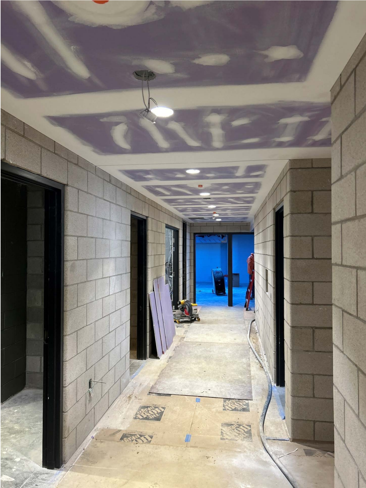
Interior Progress on 2-24-26. Ceilings drywalled and sanded.
