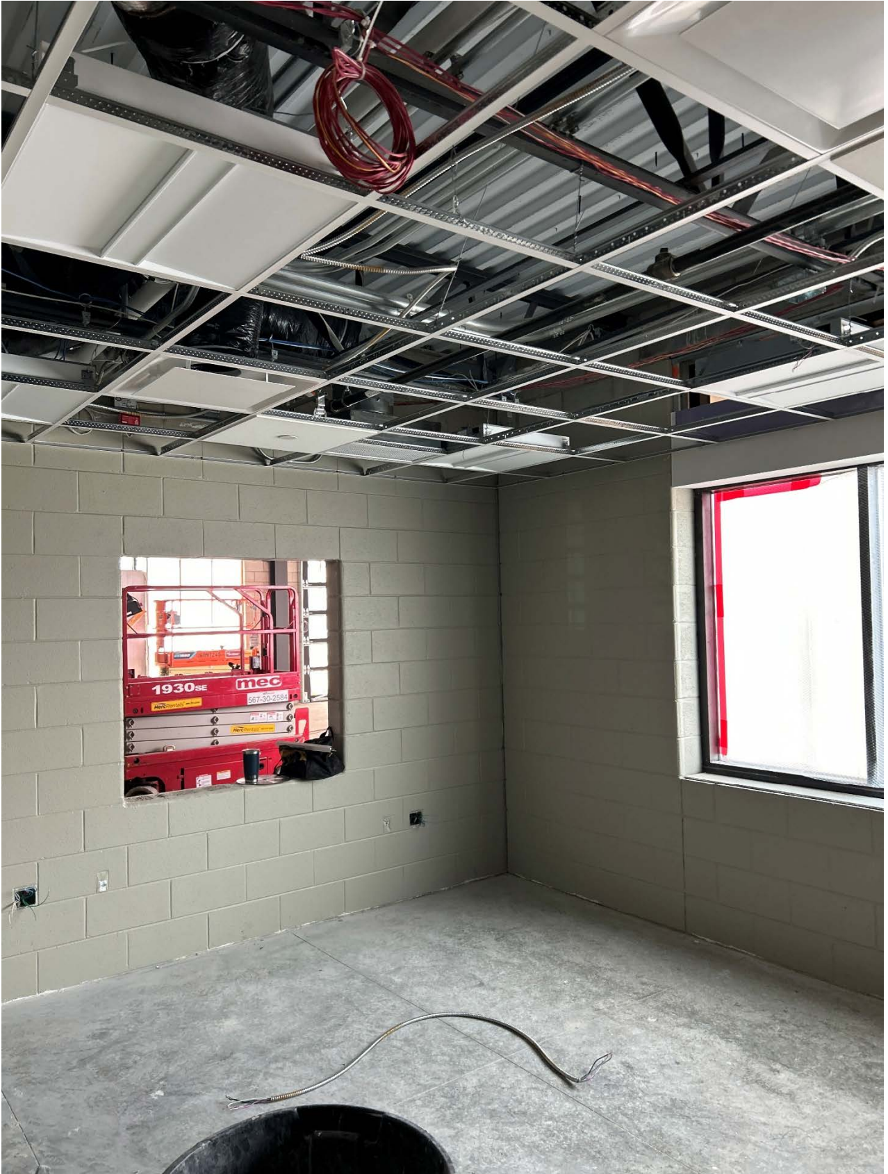
Interior progress on 2-24-26. Office with first coat paint, aluminum windows and lay-in ceiling.
