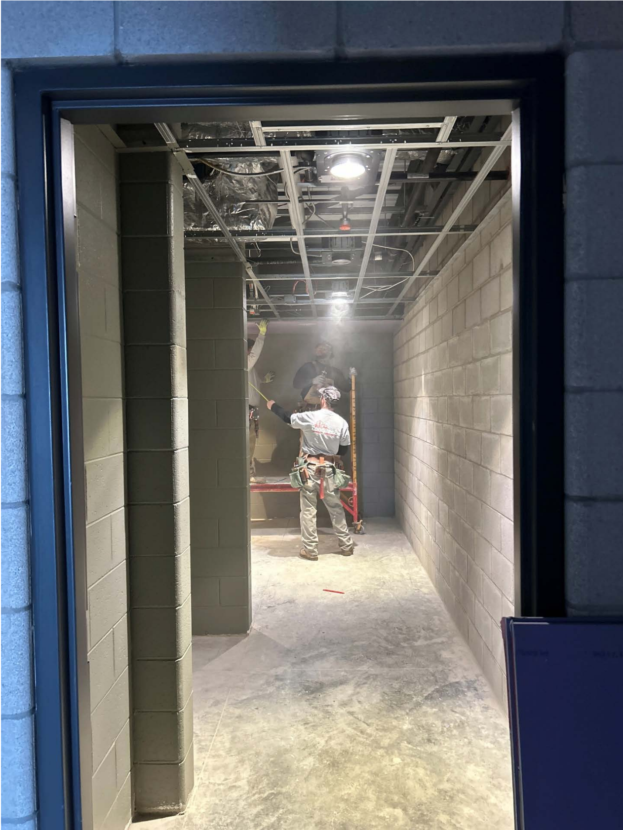
Interior progress on 2-17-26. Drywall hanging in bathrooms.
