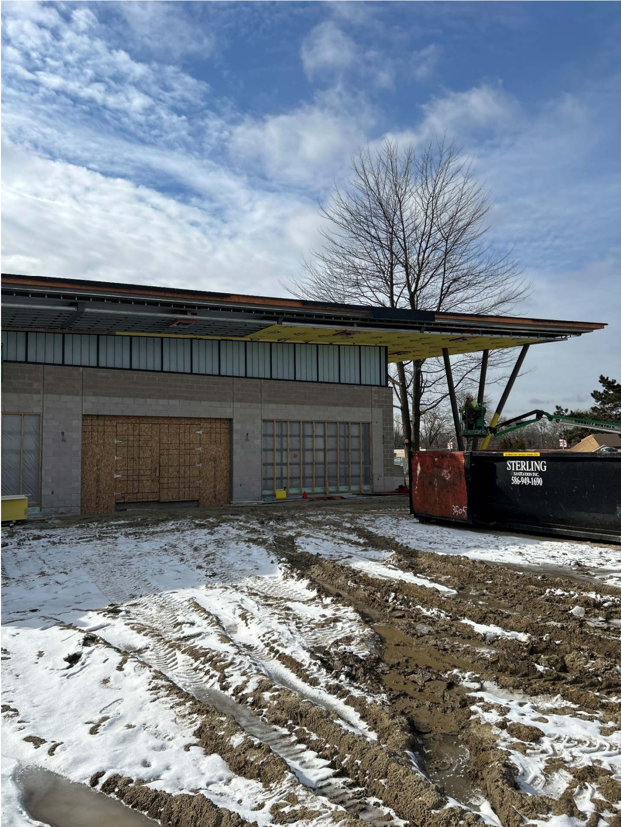
Exterior Event Hub progress on 2-24-26. Densglass substrate started on soffits.
