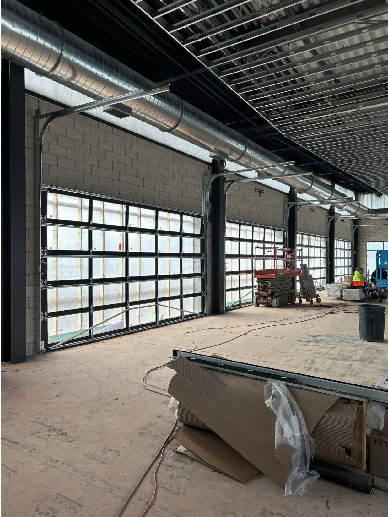
Event Space progress on 2-24-26. Overhead doors are hung. Installation ongoing. Ceiling ready for metal cladding.
