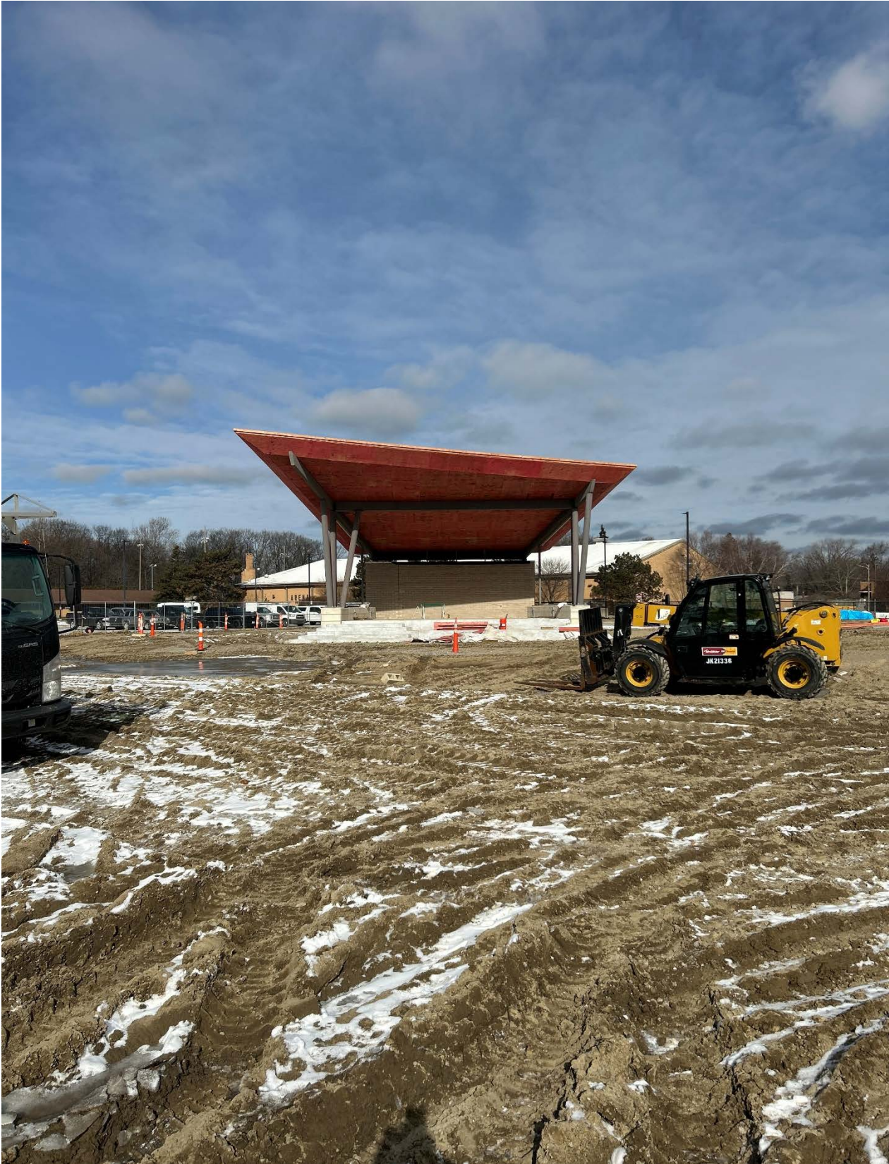
Bandshell progress on 2-24-26. Plywood ceiling substrate installed and ready for air and vapor barrier.
