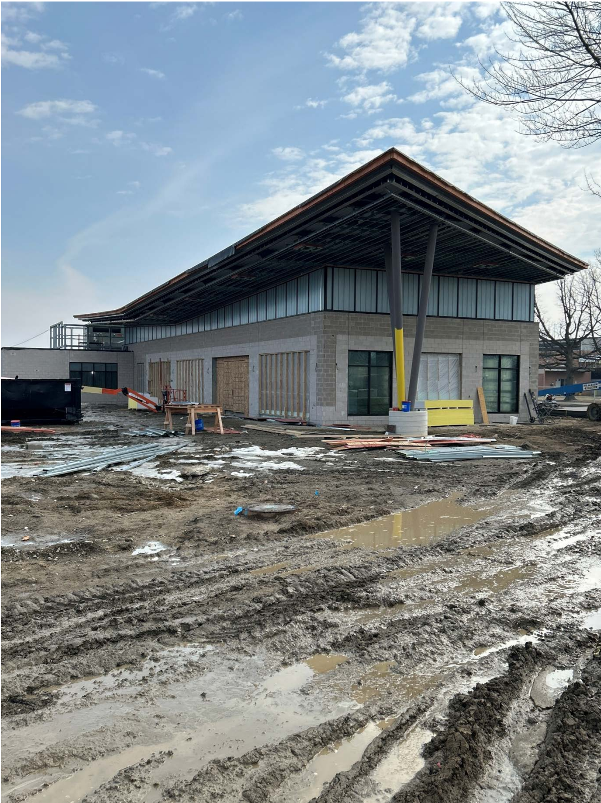
Event Hub Progress on 2-17-26. Translucent panels installed. Aluminum windows installed. Exterior soffits ready for substrate.
