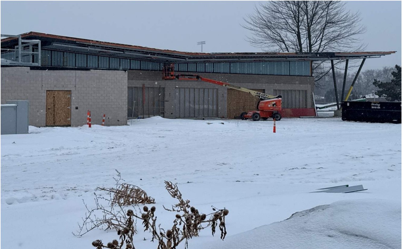
January 30 – Event Hub status – Translucent panel installation
