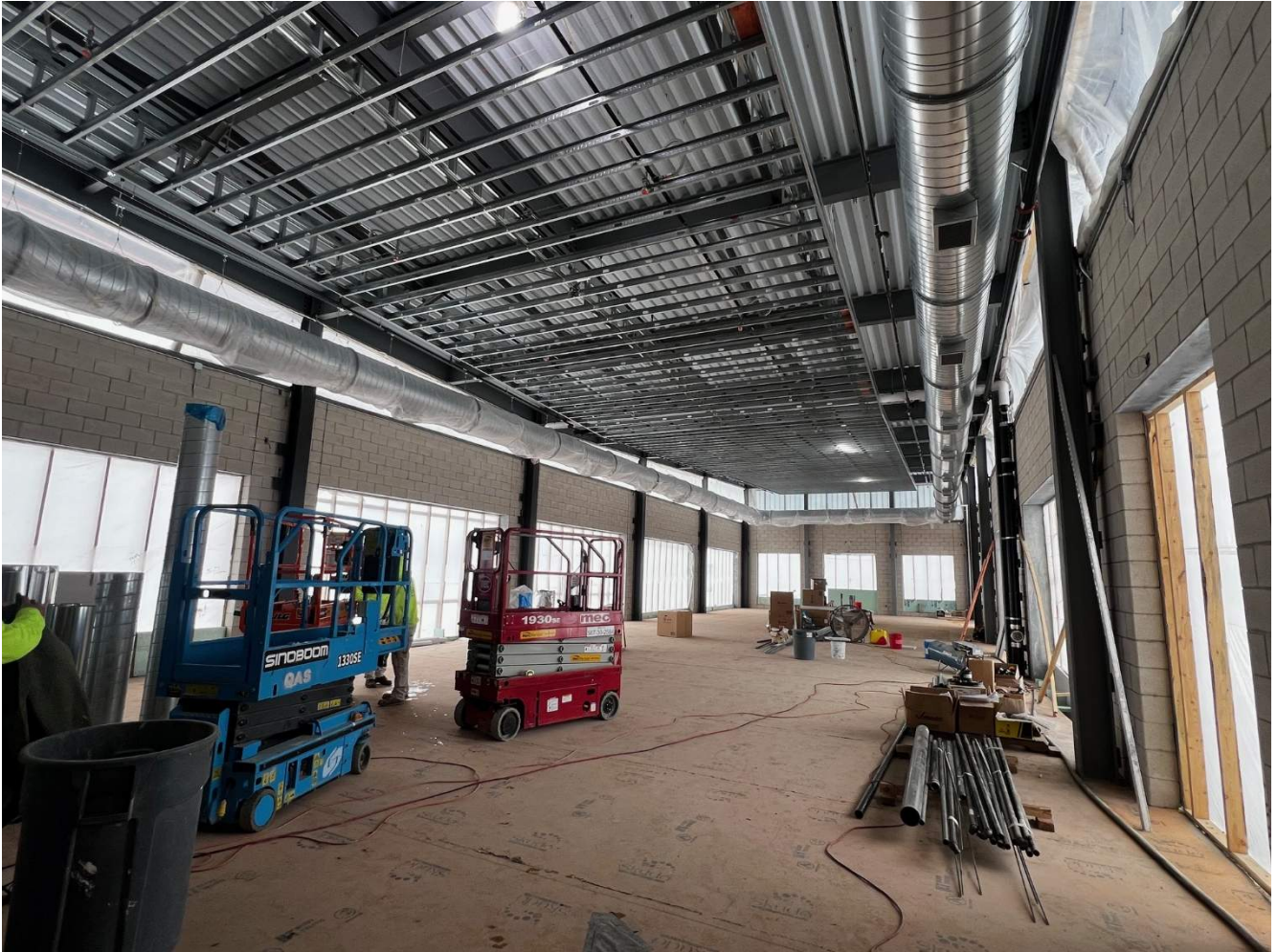
January 30 – Spiral duct complete – with diffusers
