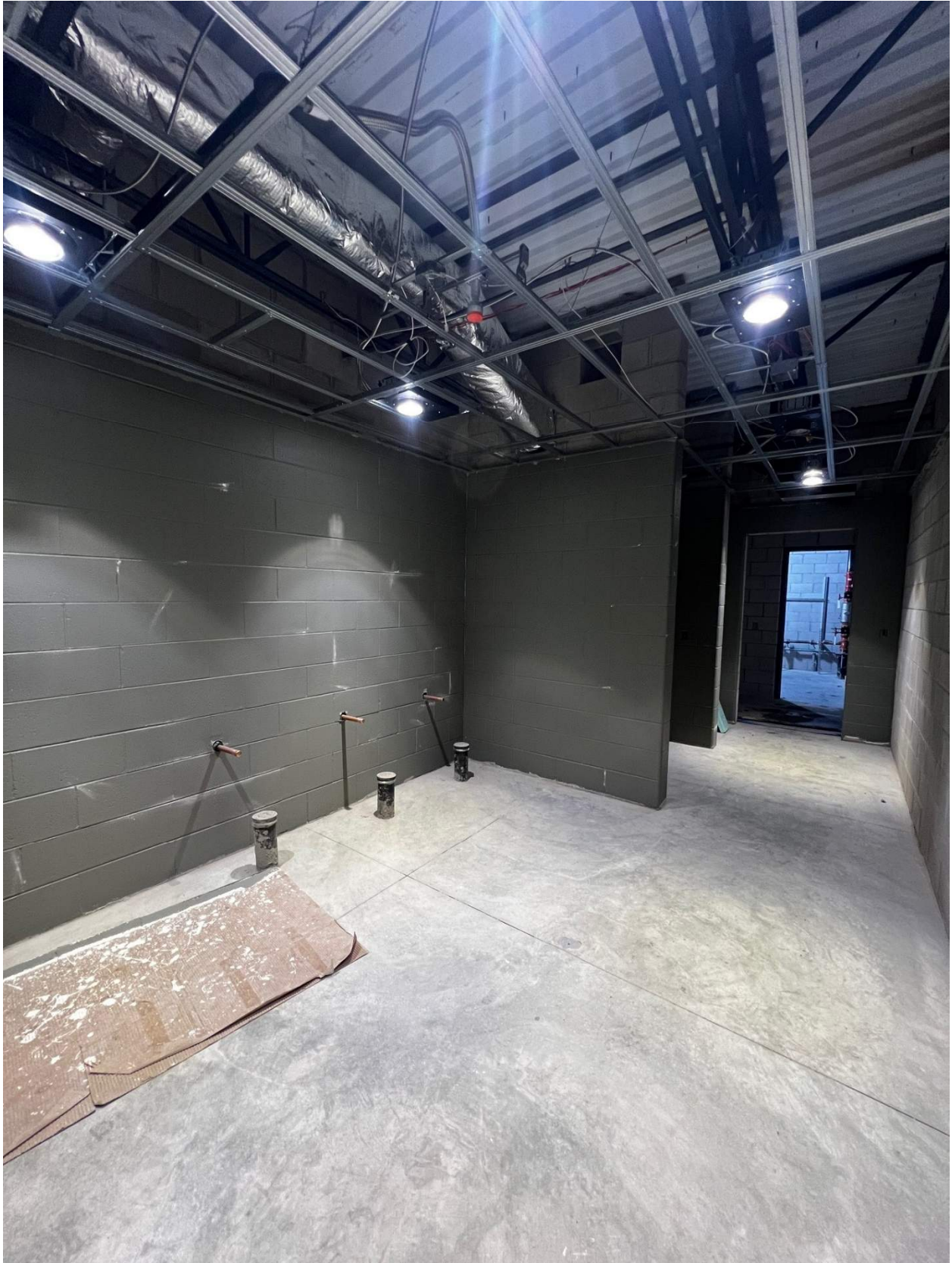
January 30 – Women's restroom – 1 st coat of paint, lighting, & ceiling framing complete
