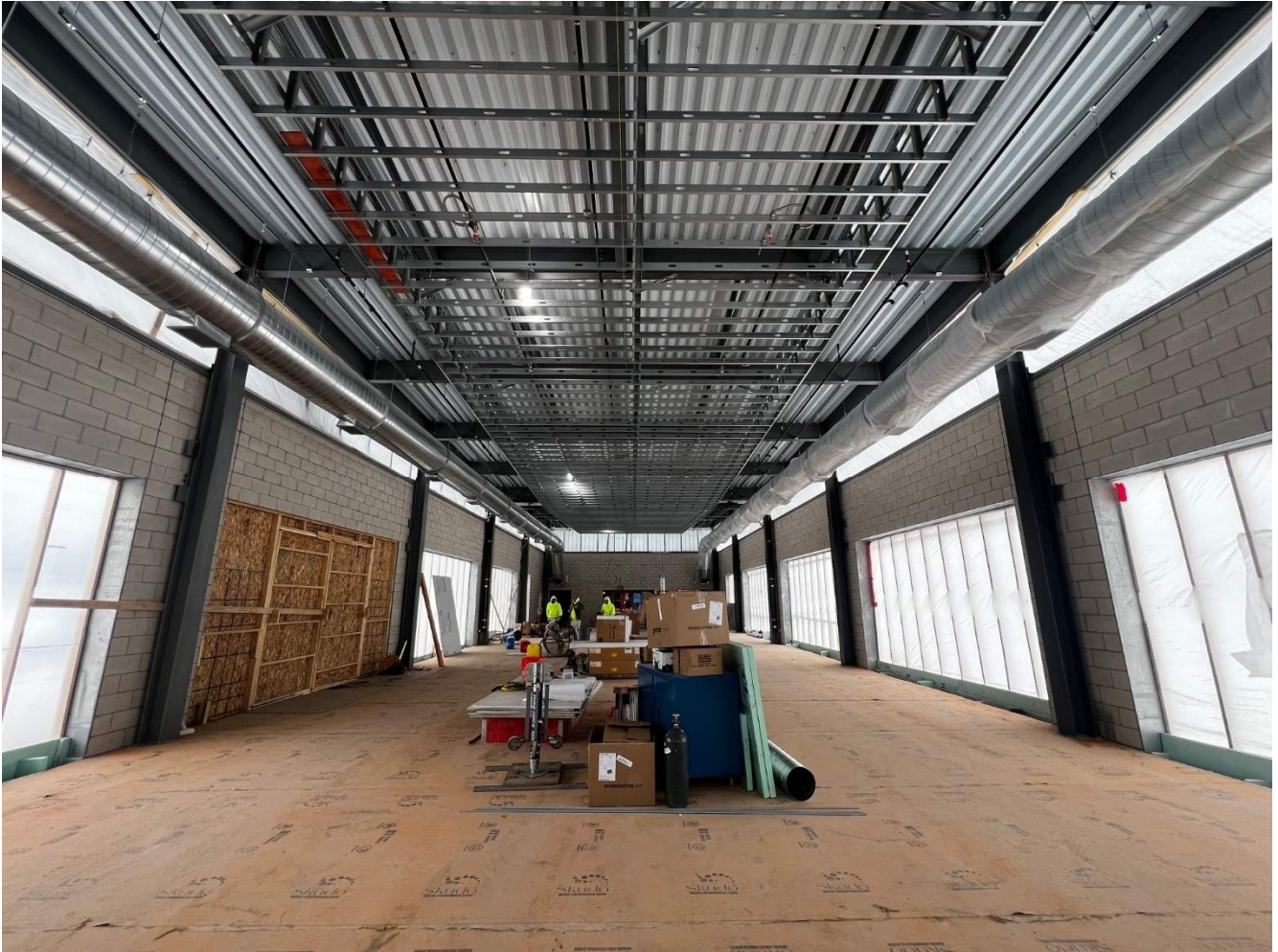
January 30 – Linear metal ceiling framing substantially complete
