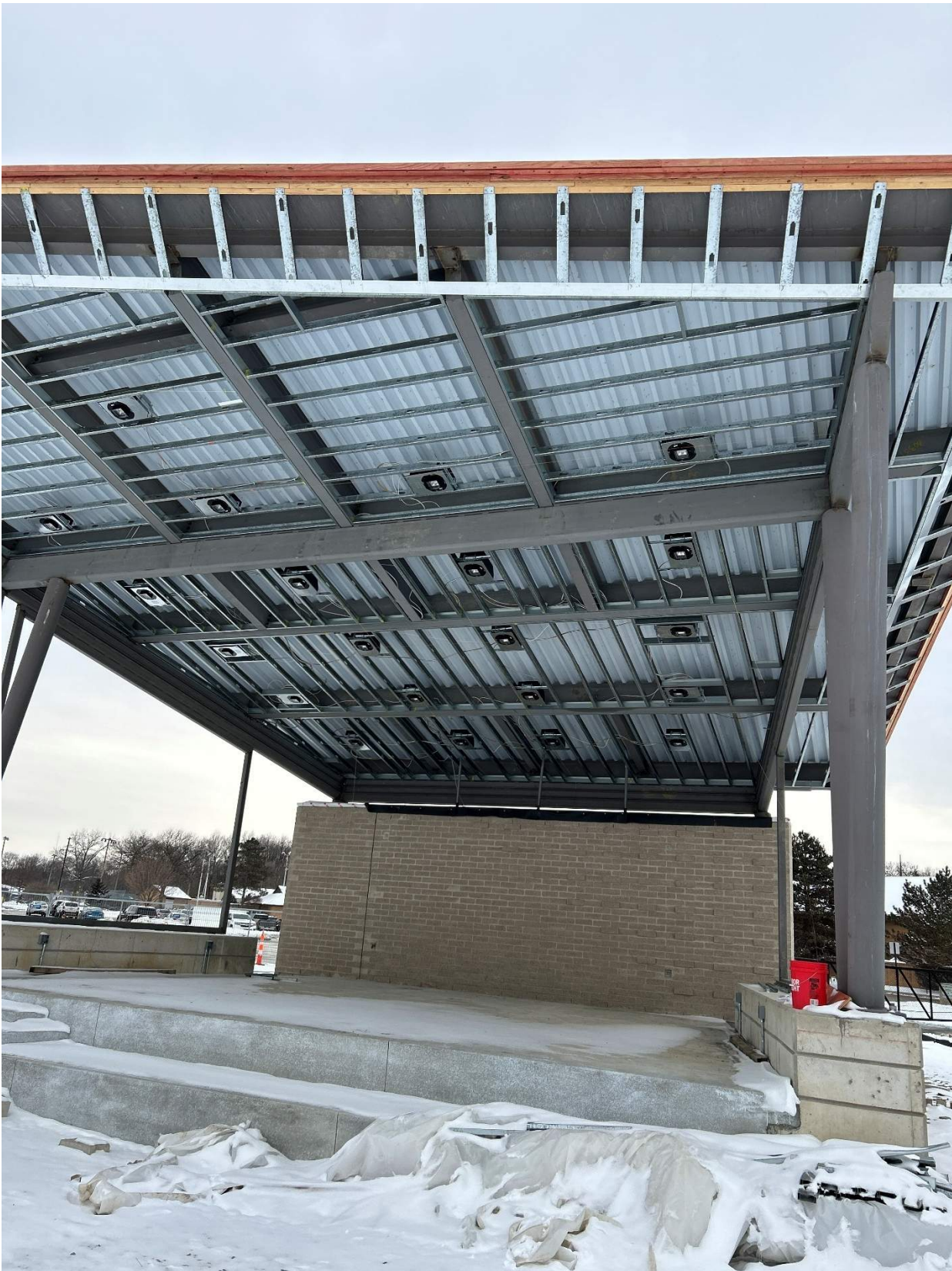
January 30 – Bandshell progress – soffit framing and lighting complete
