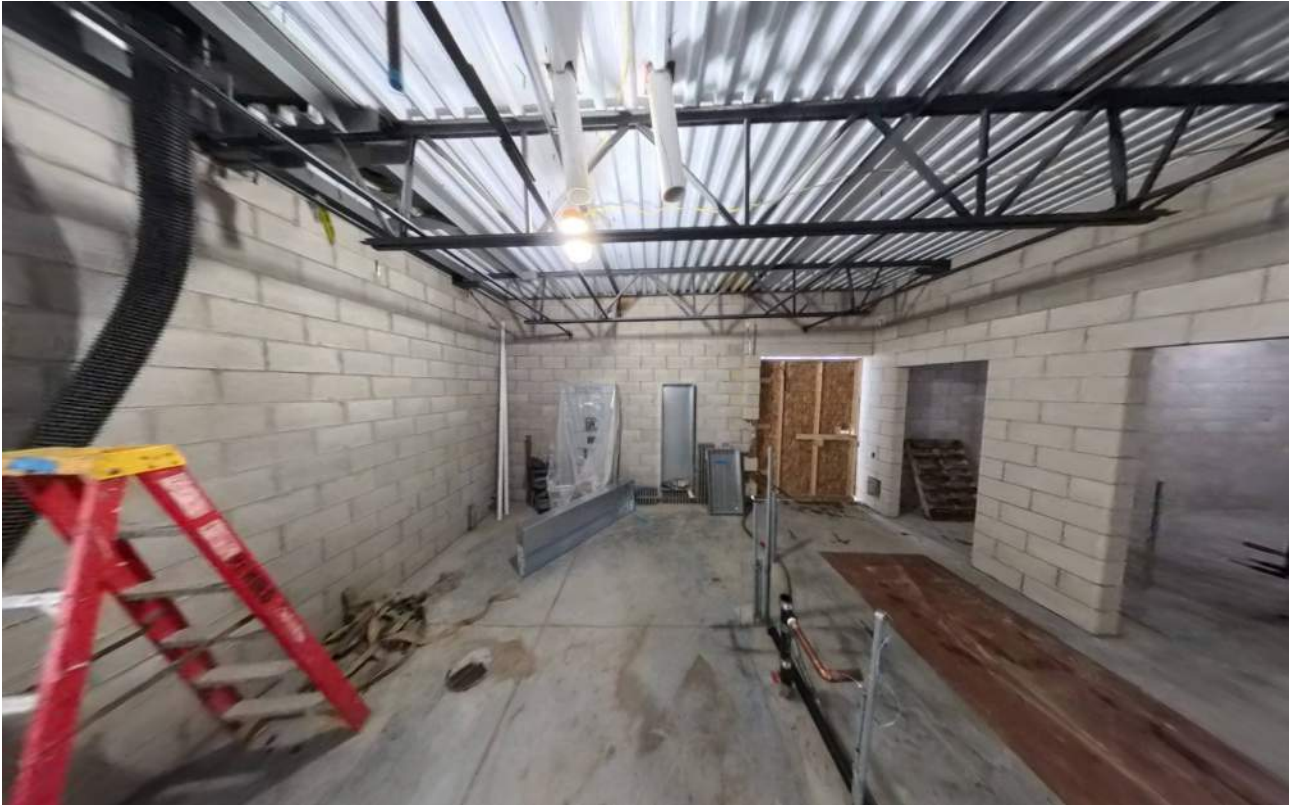
December 1 – Electrical main distribution panel and sub panels being set in Mechanical Room
