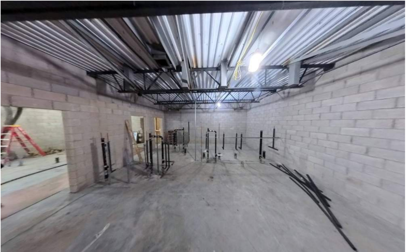
December 1 – Rough sanitary plumbing in bathrooms
