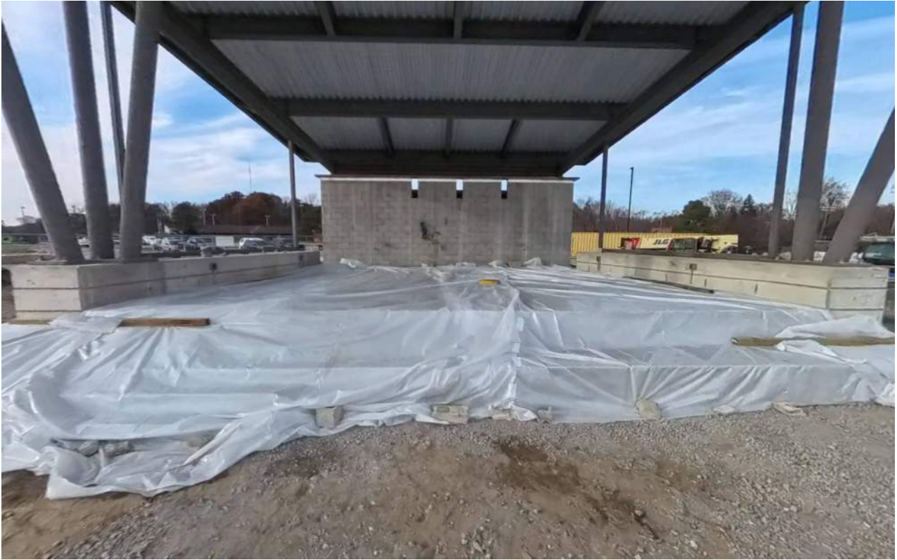
November 21 – Bandshell concrete covered for winter protection
