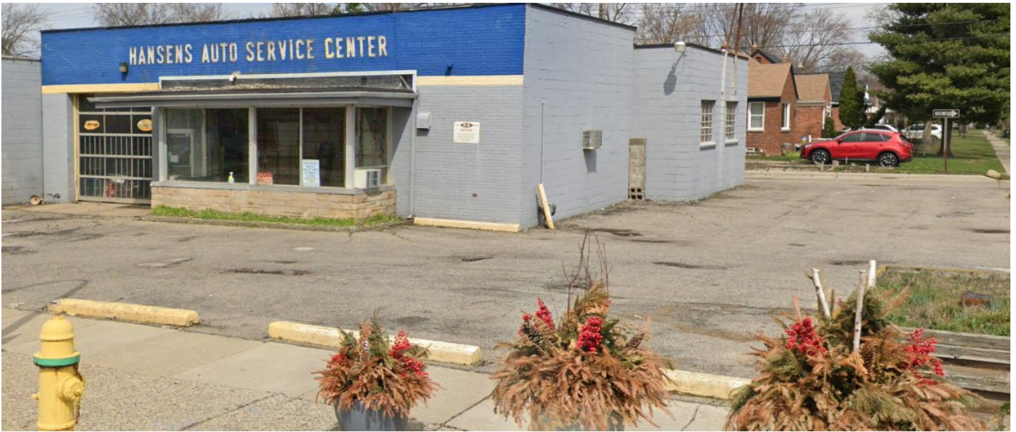
Before 8210 Nine Mile Road
