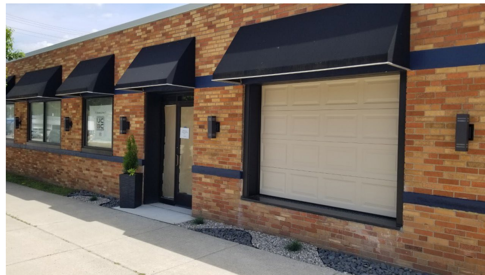
14401 Eleven Mile – Unexpected Craft Brewing Company
