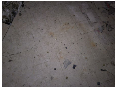
View of 9"x9" Vinyl Floor Tile (10A-B)
