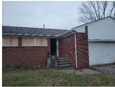
Front View of Subject Structure
