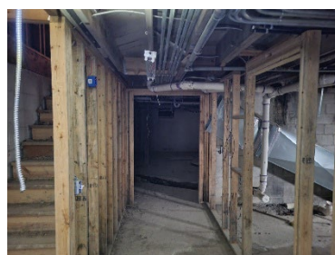
View of Basement
