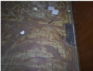
View of 9"x9" Vinyl Floor Tile (4A-B)
