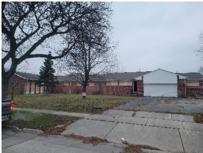
View of Subject Structure
