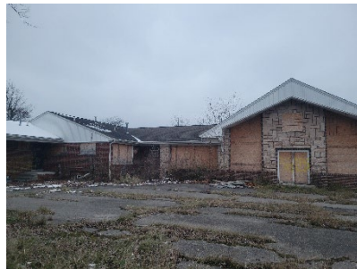
Right View of Subject Structure
