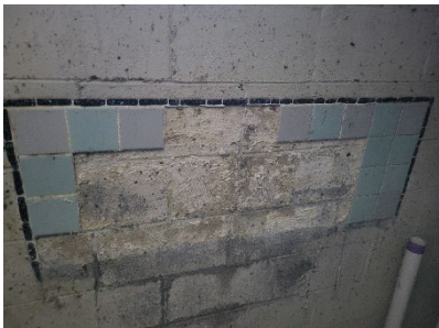
View of Ceramic Tile Bedding (13A-B)
