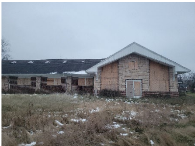
Back View of Subject Structure
