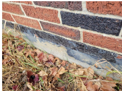
View of Foundation Sealant (20A-B)
