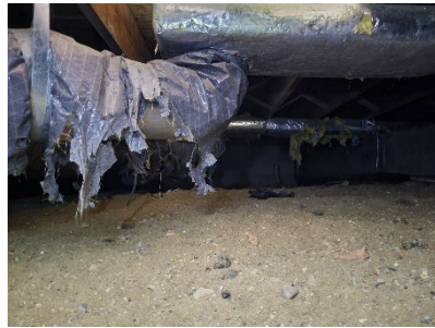
View of Crawl Space
