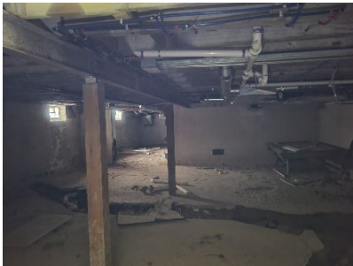
View of Basement
