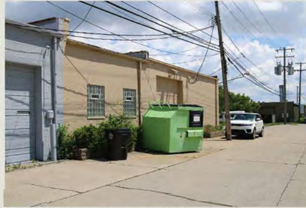
Trash receptacle without an enclosure in the alley
