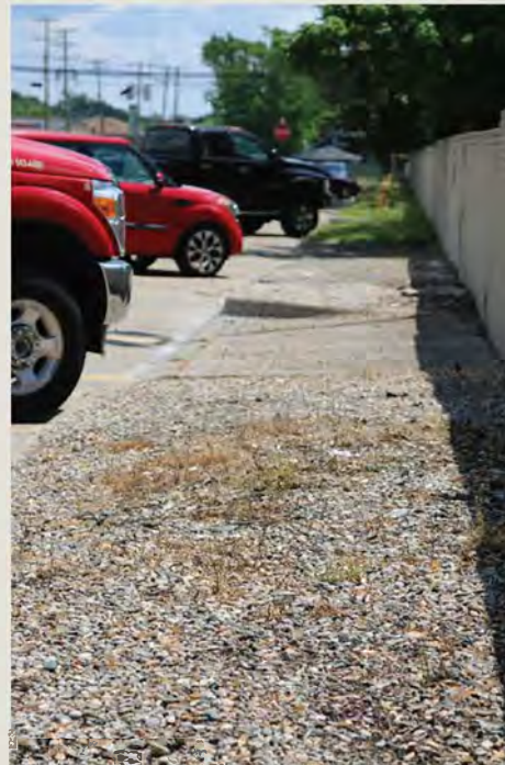
Unsafe space and curb along the wall
