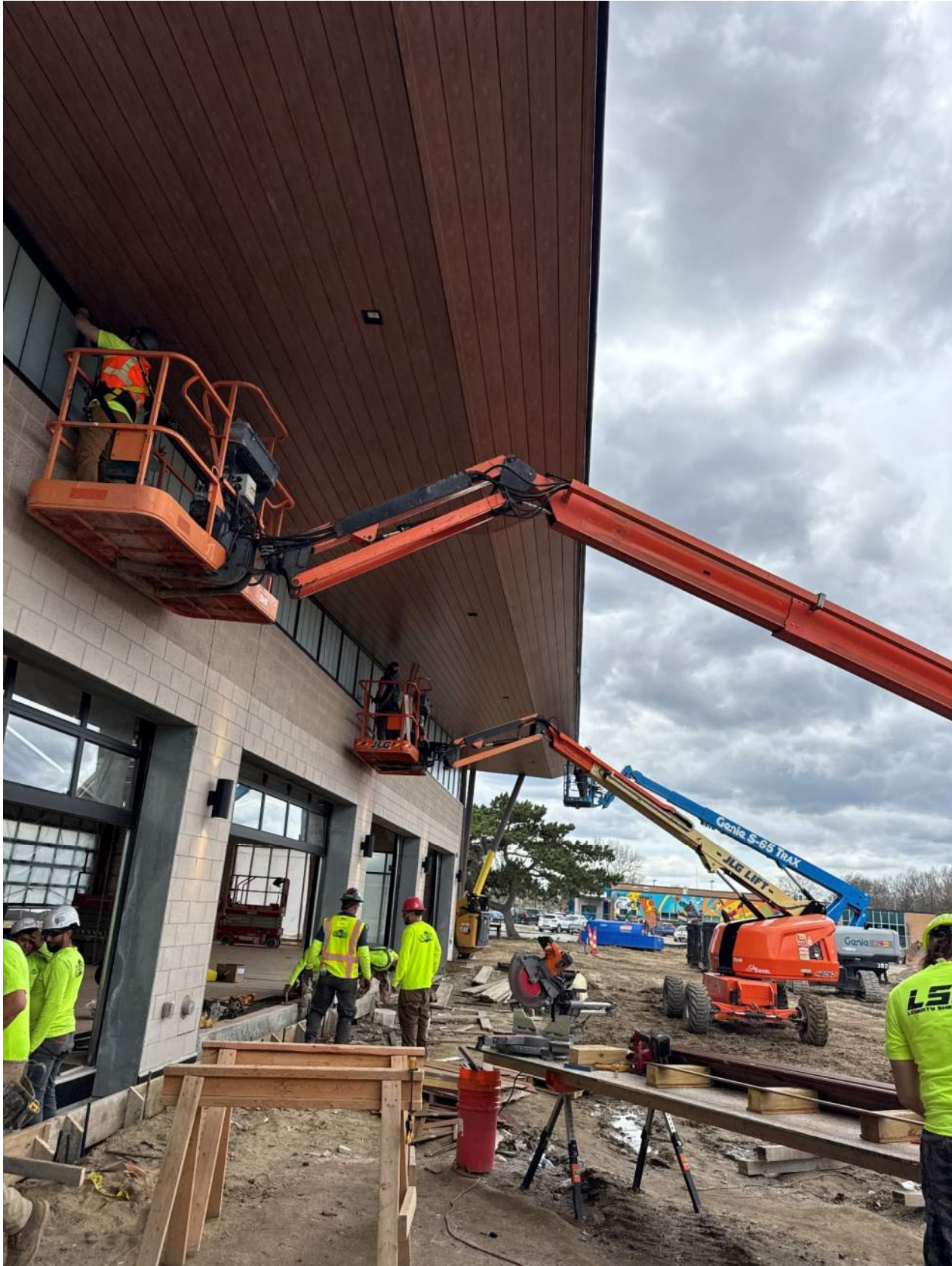
4-14-2026 Exterior metal soffit work and concrete flatwork preparation at Event Hub
